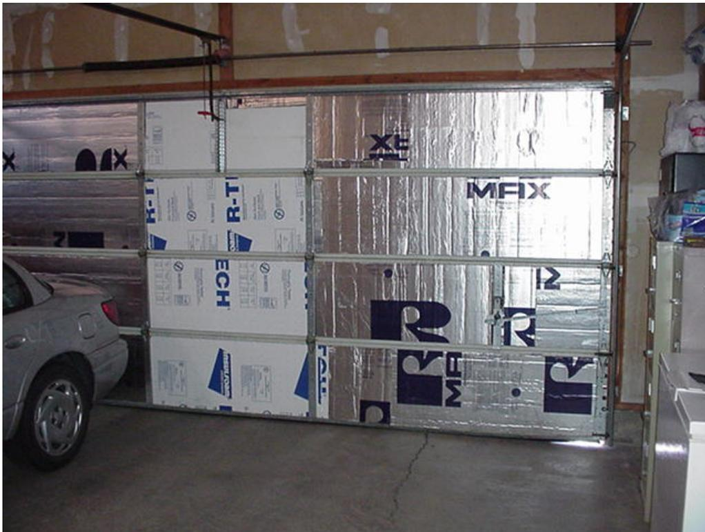
FIGURE 2 The foil-backed insulation cuts cleanly with a razor knife, whereas the compressed (white) styrofoam tended to crumble into messy electrostatic crumbs. The insulated garage is much more comfortable both winter and summer, and helps moderate the temperature of the attached living space.
