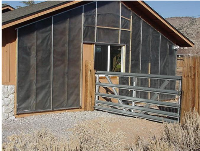
FIGURE 1 Solar air heater on the south side of a garage. Approximately 450 cfm of cool air is drawn into the solar collector, heated, and then blown into the house at approximately 120°F at noon on a sunny winter day when the ambient temperature might be 45°F.
