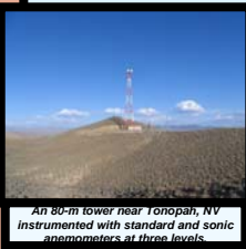
An 80-m tower near Tonopah, NV instrumented with standard and sonic anemometers at three levels.
