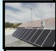
Roof installation at a school in Carson City, NV
